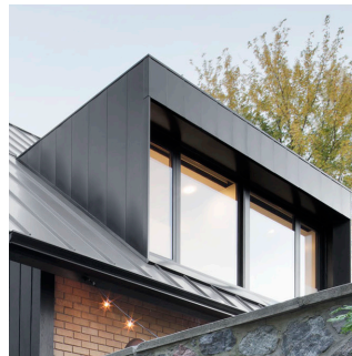
Shed dormer with a contemporary treatment. Résidence Closse, Nature Humaine, Canada
