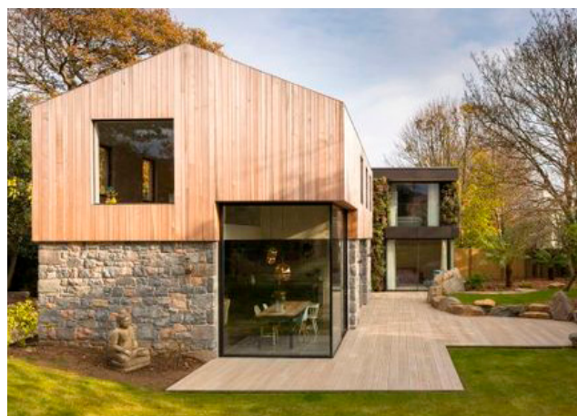
4. The siting and volumetrics of this house were calculated to preserve the root systems of protected trees. In addition, the L-shaped volume makes the structure less imposing.
