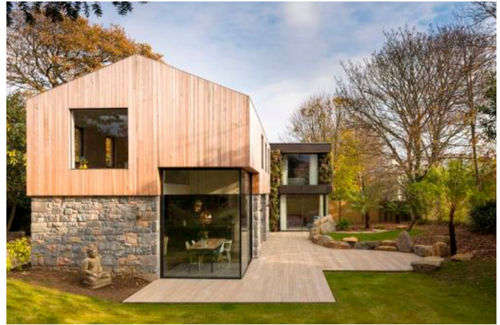
1. Ground floor clad in masonry, upper floor in lightweight wood cladding. The Glade, DLM Architects, United Kingdom
