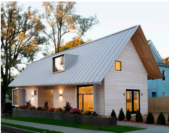
4. Steep double-pitched roof, distinctively shaped and featuring a shed dormer. Homeless shelter, Yale University, United States
