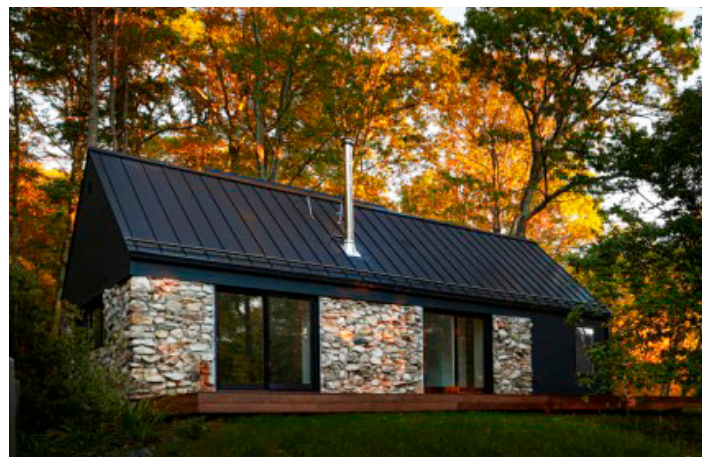
4. Ground floor clad in masonry, upper floor clad in lightweight metal cladding. Old Stone House, Takatina Design, United States
