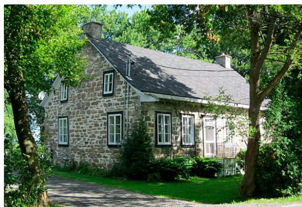
1. Eustache-Rouleau House, built in 1836. 294 Chemin de Senneville
