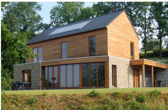
3. Ground floor clad in masonry, upper floor in lightweight wood cladding. Bioclimatic house, Eric Lambotte Benoît Straeten, Belgium
