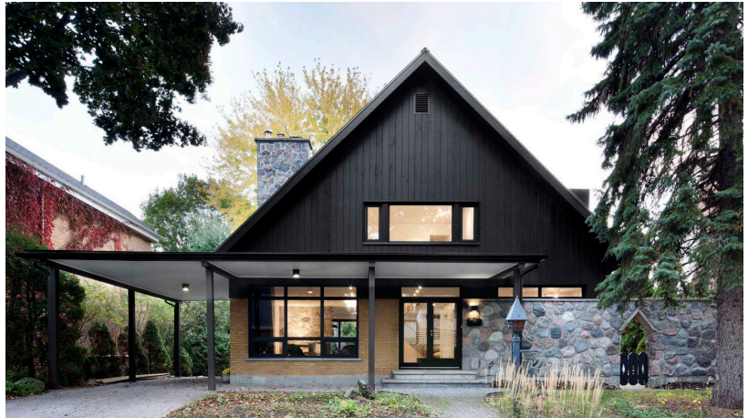
1. Steep double-pitched roof forming a gable in front. Résidence Closse, Nature Humaine, Canada
