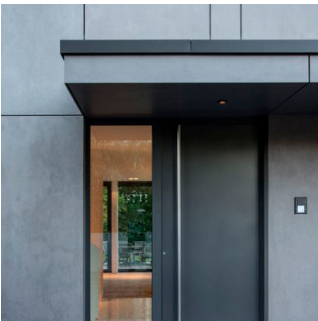
Awning with smooth fascia and flashing. Door without mouldings. Monolithe anthracite, E2 arch., Germany
