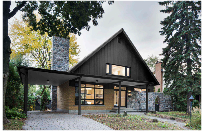
3. Contemporary renovation of a house influenced by American vernacular architecture. Résidence Closse, Nature Humaine, Canada
