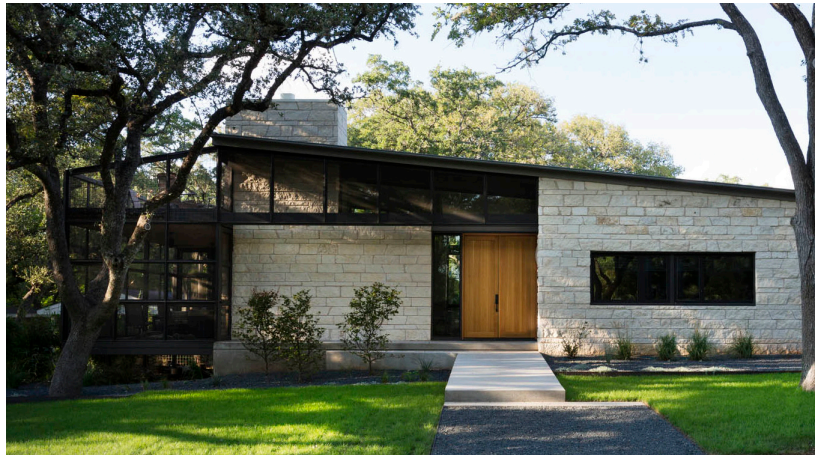
3. Single-pitch roof with a gentle slope. River Road, Cuppett architects, United States
