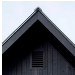
Roof peak with minimalist fascia and no ornaments. Vent the same colour as the cladding. Résidence Closse, Nature Humaine, Canada
