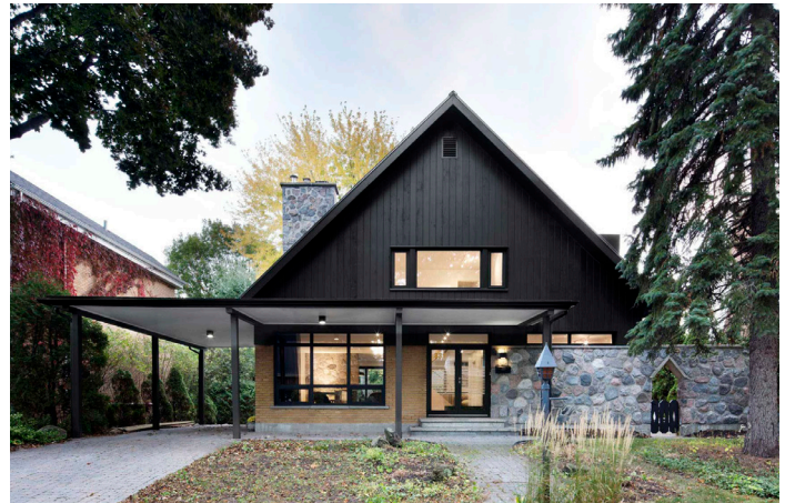
2. Masonry and fieldstone ground floor, upper floor in lightweight wood cladding. Résidence Closse, Nature Humaine, Canada
